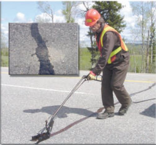
**CRF<sup>®</sup> Restorative Seal** is a petroleum oil and water cationic emulsion. Unlike standard asphalt emulsion, CRF<sup>®</sup> does not harden or "dry out" Designed as a one component emulsion that effectively repairs cracks in concentrated form, CRF<sup>®</sup> provides a excellent pavement restorative seal when applied in diluted form.
