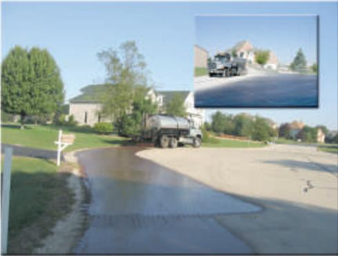
CRF<sup>®</sup> provides pavement rejuvenation as well as sealing the pavement surface, unlike standard asphalt emulsion that hardens and becomes brittle. CRF<sup>®</sup> was designed to be a corrective maintenance product that effectively repairs cracks as a "cold pour crack filler" in concentrated form and provides a pavement "restorative seal" when applied in diluted form.
