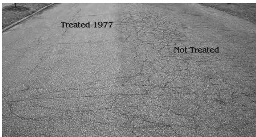
After 32 years, 2009 photo shows performance of 1977 maltene-based rejuvenator emulsion-treated pavement in Cleveland, Ohio
