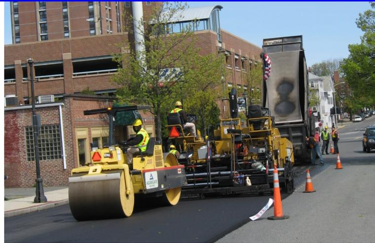
Thin-lift asphalt pavement preservation treatment incorporating warm-mix technology and polymer-modified emulsion is demonstrated on a Salem, Mass., arterial.
