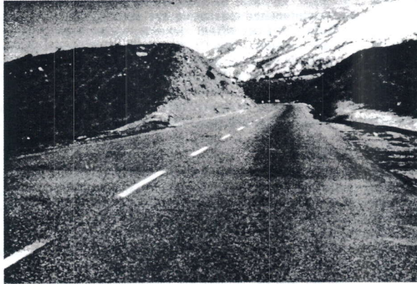
Figure 26. White Wolf Grade section six months after treatment: treated lanes in background; untreated lanes in foreground.
